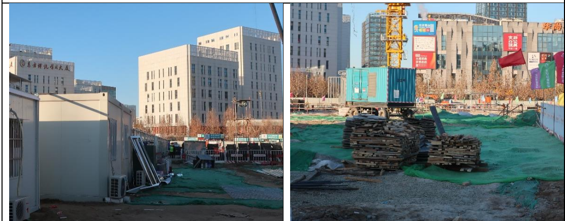
施工临建区临时覆盖 (2021.12)
