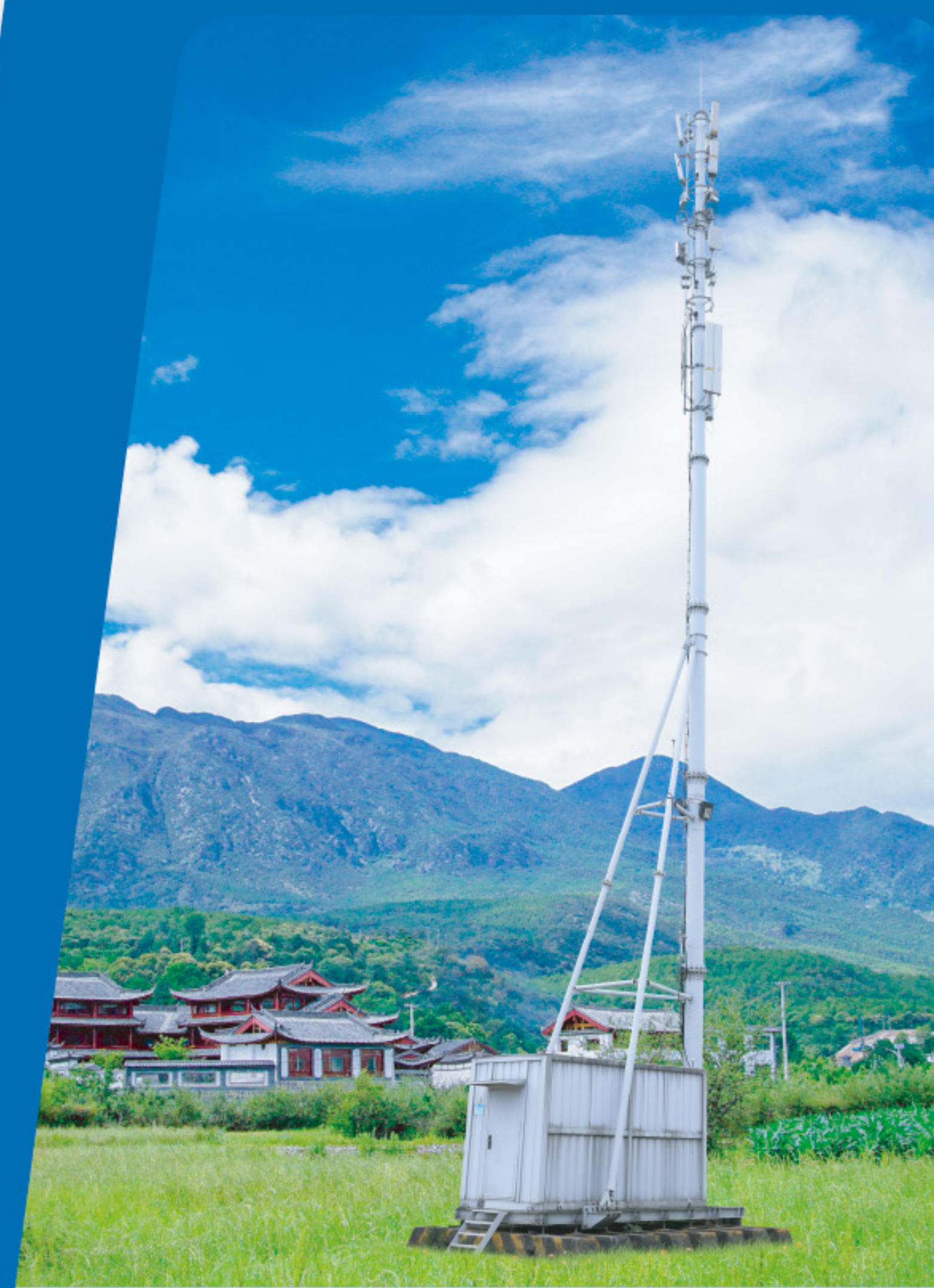
Fast build Base Station
